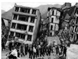
Building collapse in Nepal
